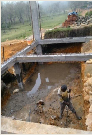
UNDER GROUND SUMP 35000LTRS CAPACITY, LOCATION: KODAIKANNAL
