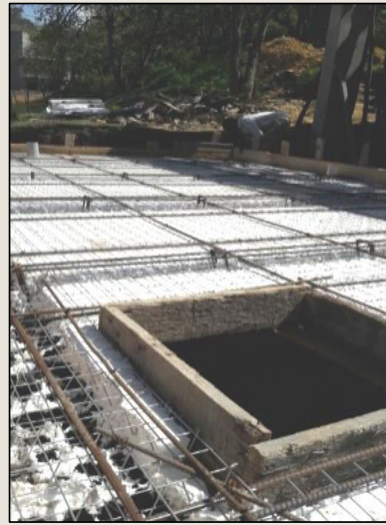
UNDER GROUND SUMP 35000LTRS CAPACITY, LOCATION: KODAIKANNAL
