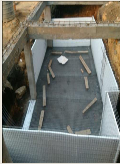
UNDER GROUND SUMP 35000LTRS CAPACITY, LOCATION: KODAIKANNAL
